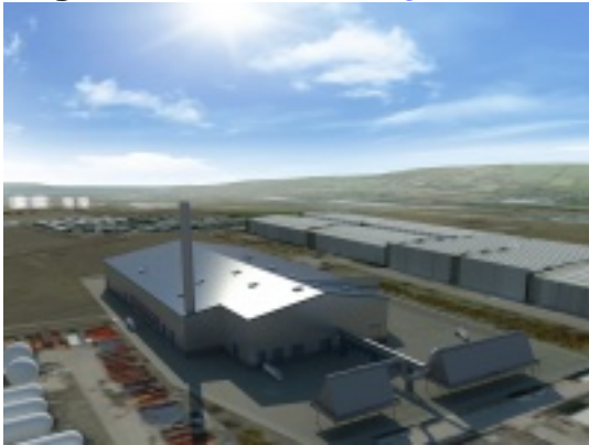
Waste-to-Energy Gasification Plant
